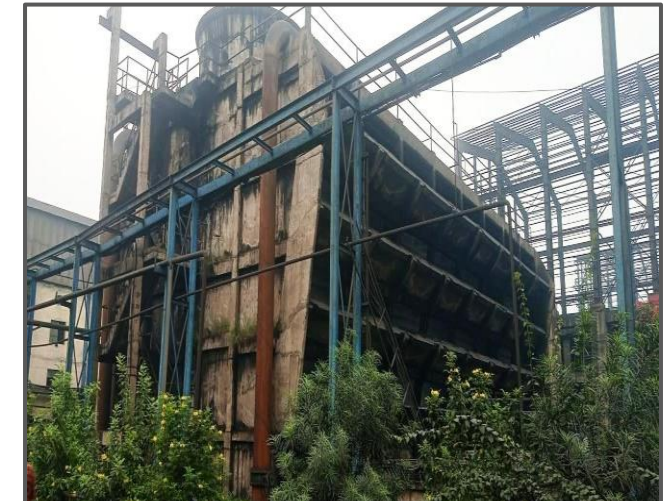
Neutralizing Tank
