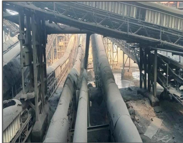
Conveyor For KILN
