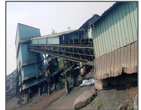
Screening House for Coal Circuit
